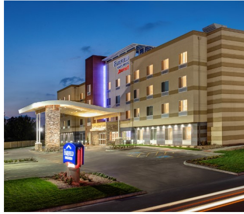
Fairfield Inn & Suites by Marriott-Terrell, Texas
